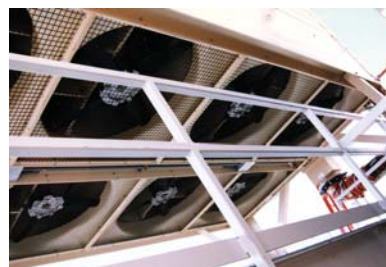
Modular Cooling Tower with bottom mounted mechanical equipment
