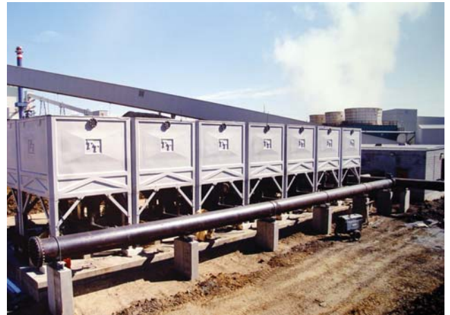
An early Modular Cooling Tower constructed of hand-laid-up fiberglass
